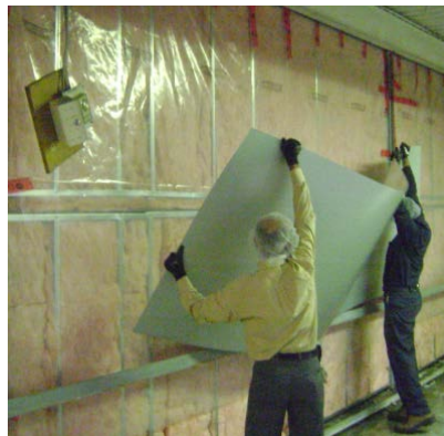
Insulation of R-10 insulation at the inner portion of the dock at Thermoforming Plant 1
